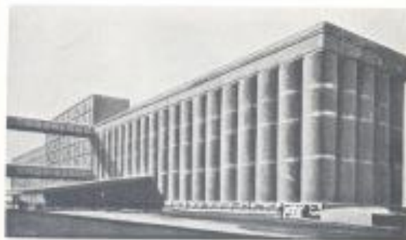
CHADIAN DRAIN TOWER AND ELEVATORS
